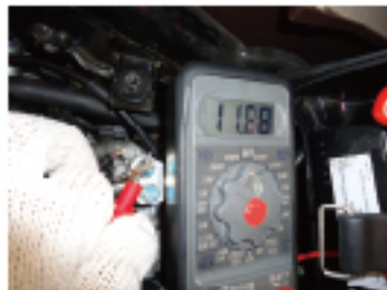
6. TURN ON THE SWITCH AND CHECK WHICH WIRE IS (+).
