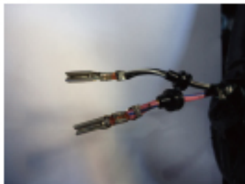
5. FASTEN TWO WIRES AS ABOVE PHOTO.
